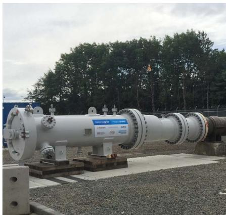
GRAID launch vessel connected to the NTS.
