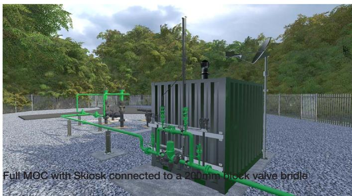
Full MOC with Skiosk connected to a 200mm block valve bridge
