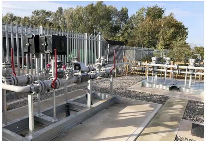
The picture above shows the meter skid (foreground) and filter skid (background) enhancements installed at Eakring
