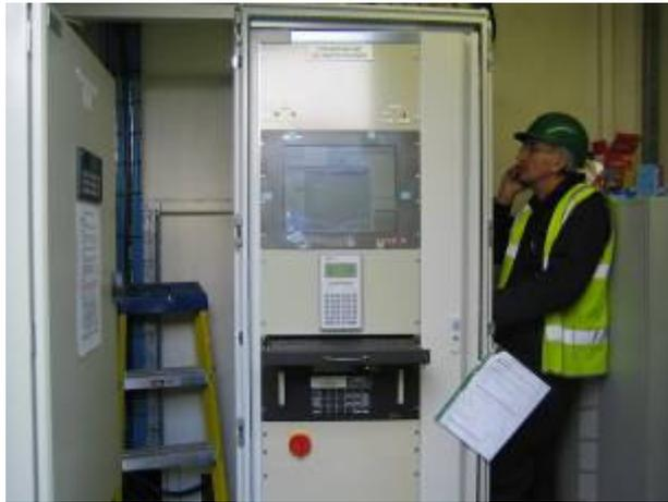
Figure 2. New flow computer and supervisory system panel with upgraded flow computer, supervisory system and new gas chromatograph controller, 2350A
