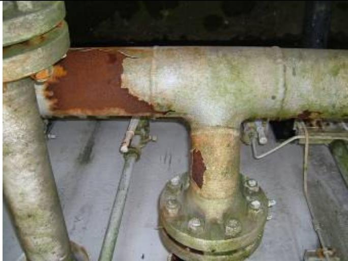
The outcome of this project will be the identification of two coat paint systems that are compatible with existing materials. Maintaining the existing coating system, rather than effecting its complete removal and replacement, will provide a more cost effective solution to maintenance painting.
